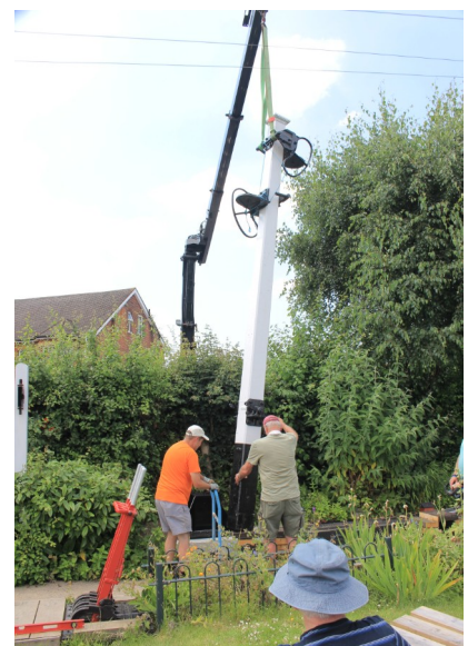
Above: the HIAB returns to St Albans to lift the post into its collar.
