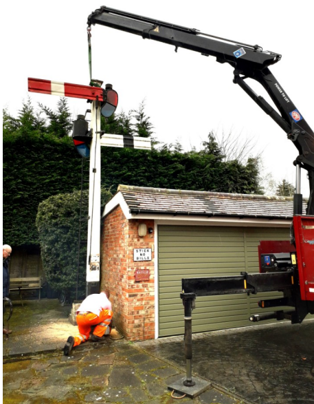
Above: the HIAB is in place in Woking and the post is being cut off at ground level. Centre top: work starts on dismantling the metal work. Centre bottom: work completed, the post is wheeled into position ready for lifting.
