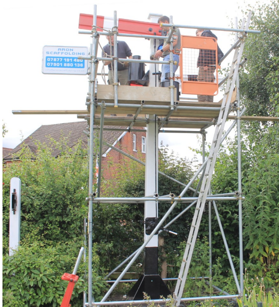
Left: the post is in place, the scaffolding erected and the assembly of the signal arms and mechanism can be completed. Above: the view of the Box from the scaffold tower. And finally on the right: our benefactor of the signal and funds, the late Philip Anthony Millard.
