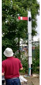
After many months of careful restoration, the North Eastern slotted post was Railway finally moved into position at the north end of the garden Wednesday 26<sup>th</sup> on July. There is still much work to do as the mechanical parts now need to be fitted as well as the finial and ladder. Then we have to work out the aeometrv of the linkage needed from the ground frame to the post to enable the signal and spectacle plate to operate.
