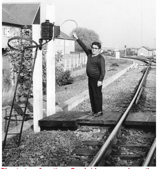
Chesterton Junction, Cambridge was where the St Ives branch left the main line. The Signalman is placing the hoop and pouch containing the single line token into the holder for collection by the driver. The lamp illuminates the hoop at night. These items are now on display in the 'box garden, donated by Andy Buckley who took the erected but the rest is as shown in the top shot.
