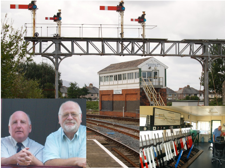
Llandudno Station Signal Box pictured in the summer of 2014. Inset left: Steve Lake on the left with fellow relief signalman from 1979, Geoff Ryland. Inset right: the interior of Steve's box, the frame only extends about half the length of the box and has a number of spare white levers.
