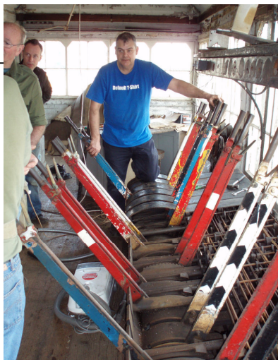
The above picture from 2007 shows members working on restoration of the frame. The interlocking can be seen to the right of the levers with the casings removed.
